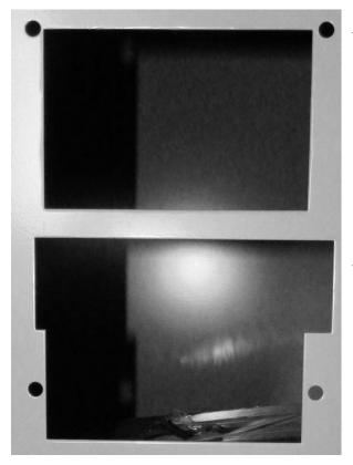
The top opening is where the cabinet air is drawn into the unit through the cooling coils. There is a temperature sensor mounted in front of the coils. Make sure it is visible after installation or incorrect operation can occur.
