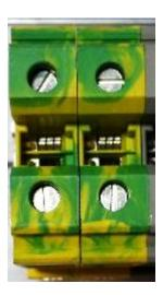
All grounds need to land at this common point including building, motor, transformer, and filter grounds. This prevents ground loops, and will limit the impedance between the grounds and noise will be channeled back to building ground.
